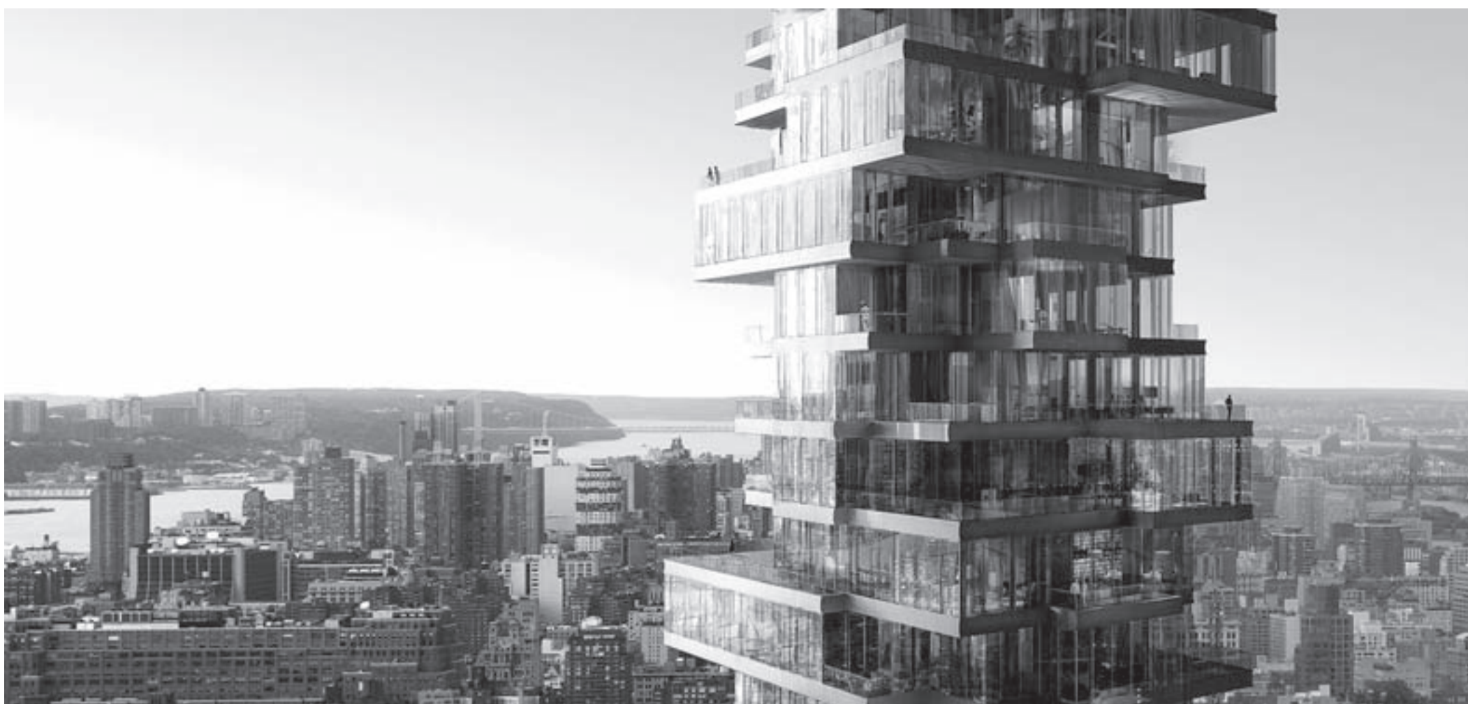
The crown of Herzog & de Meuron's tower, 56 Leonard St. in New York. Penthouses occupy full-floor glass boxes that have the effect of being staggered and shifted atop one another. HERZOG & DE MEURON
